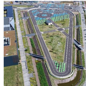
Available Transalley technopole test track Valenciennes
